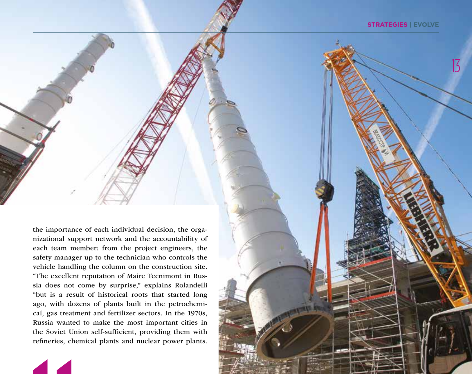
The OMSK plant, the cranes position the column on its foundation
